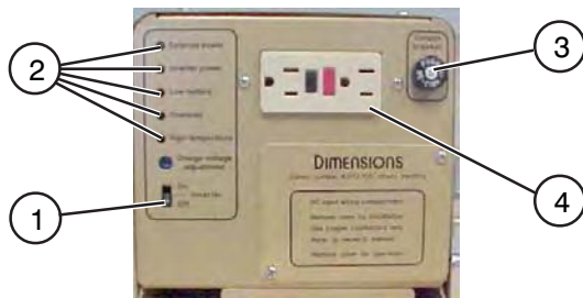
Figure 2-7. 1500W AC Inverter
